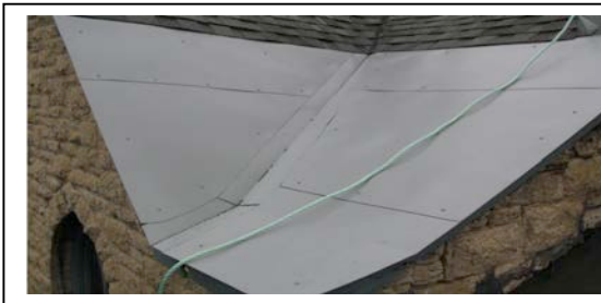
Left: Then by sheet metal to shed the snow; Centre: Ice dam on 16 December over entrance Right: Weathering effects on woodwork of the spire on Church House.
