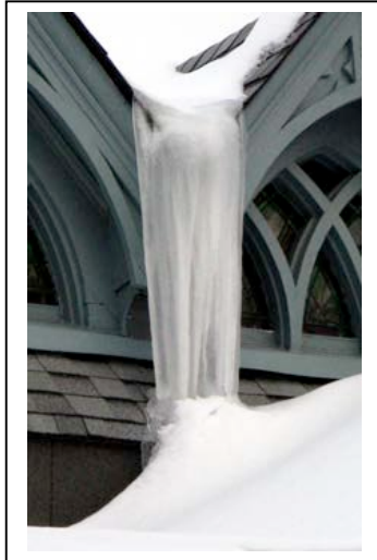
Left: Roofers working on the wall below the Stradbrook dormers; Centre: Ice dam on dormers Right: the roof by the Stradbrook entrance was covered with weather-proofing
