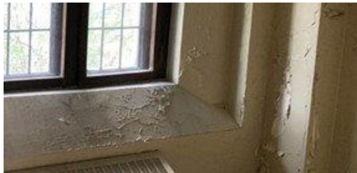
Photo showing lead paint flaking in a characteristic “alligator” pattern.
